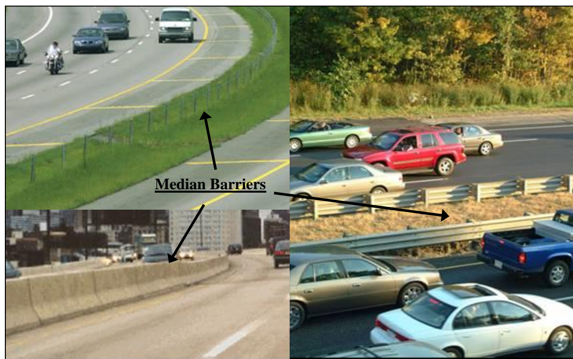
FIGURE 7 Typical Median Barriers (6).
